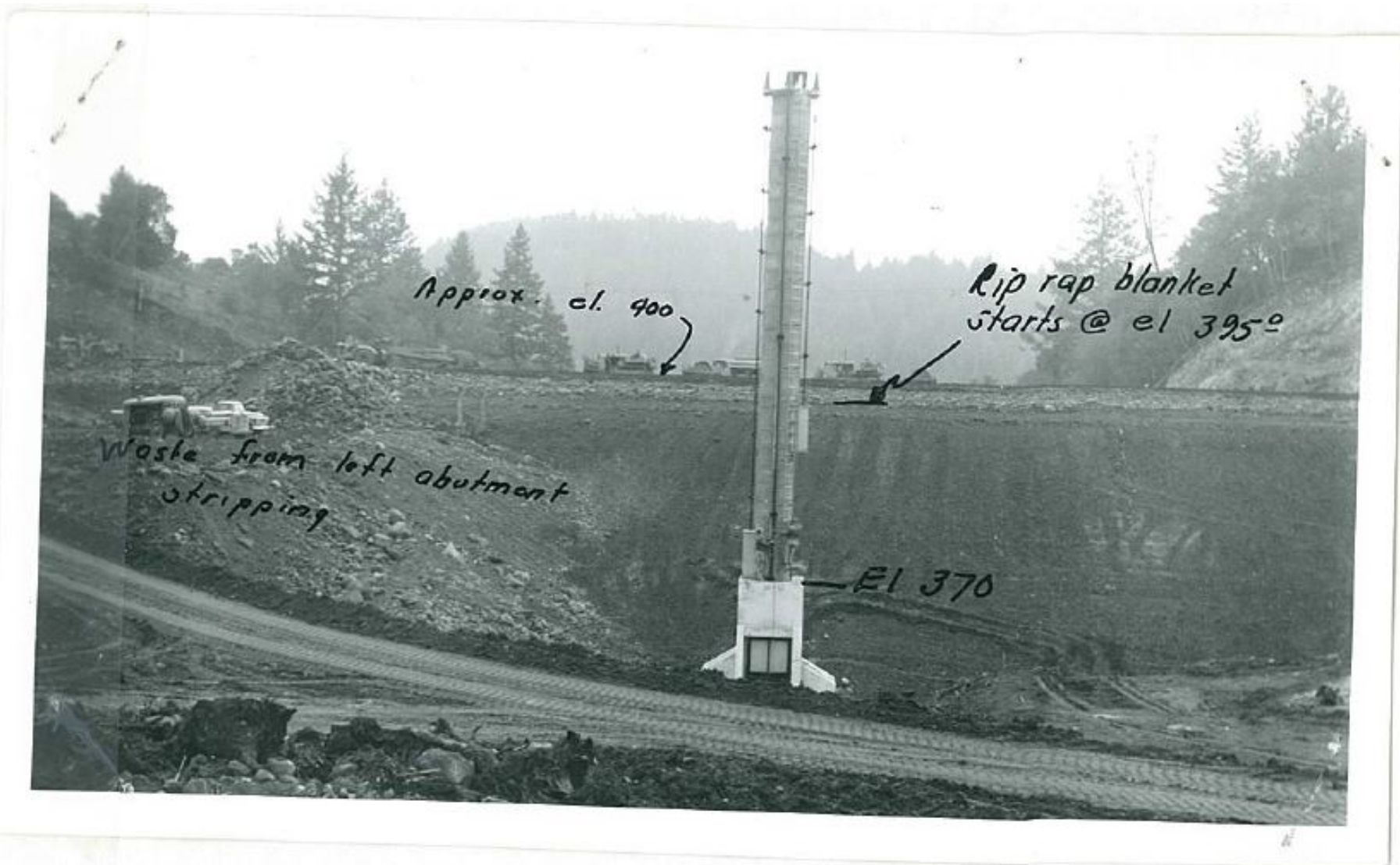
C. M. P. outlet tower installed.
