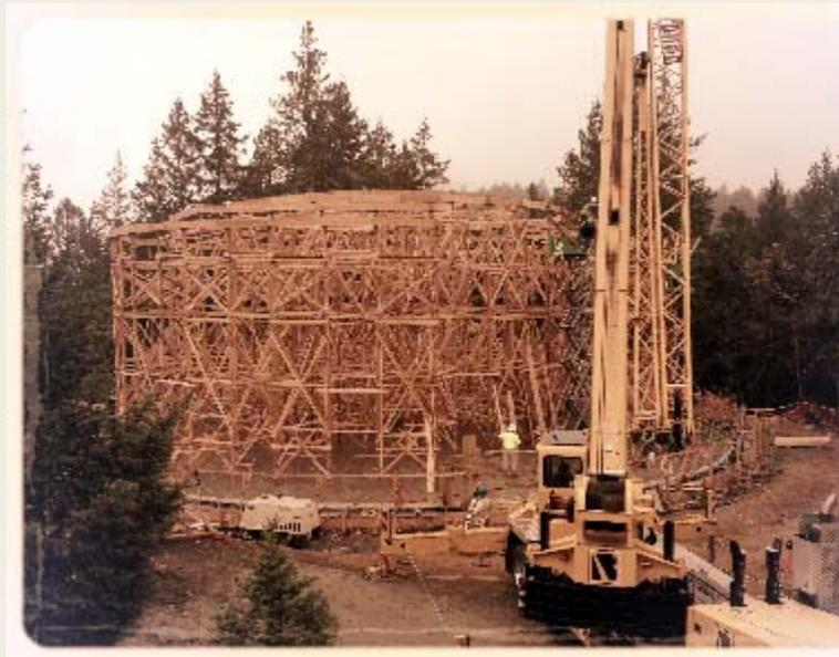
The photos above show the rising of the massive falsework framing which is necessary to provide temporary support for building the dome roofing and for the erection of the precast wall panels. Once the erection of the wall panels begin, the crane hooks onto the lifting inserts that are cast into the panels. During this tilt-up construction, the lifting crane operates from select positions to minimize the distance between panel casting beds and the final position of the panels.
