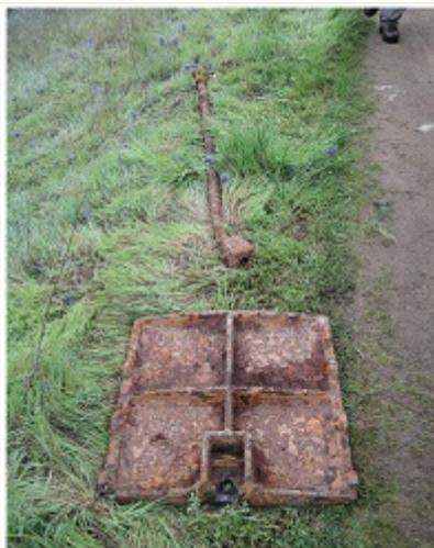
On April 4th, a four-man crew of specialist divers working beneath the surface of Bell Canyon Reservoir completed the removal of intake gate and associated appurtenances at elevation
